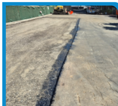
Parking lot asphalt being replaced to base layer.
