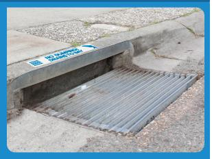
Never allow spills and leaks to enter storm drains. Federal, state, and local regulations prohibit any discharges other than rain into the storm drain.
