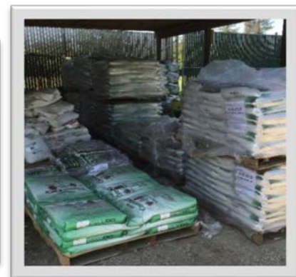
Outdoor materials stored on pallets and covered.
