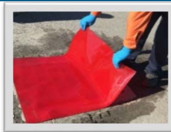
Rubber mat to protect storm drain.
