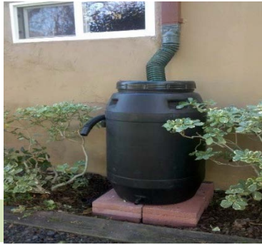
A rain barrel at a single-family home in Palo Alto
